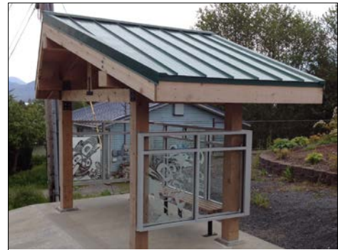
New Bus Shelter in Saxman
